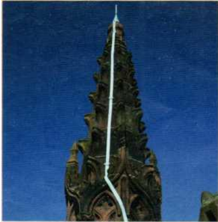
Figure 11.9 A copper lightning conductor protects a tower on a building.
