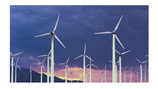
Windmill – Mechanical (wind) → Mechanical (turning blades) ) → Electrical energy
